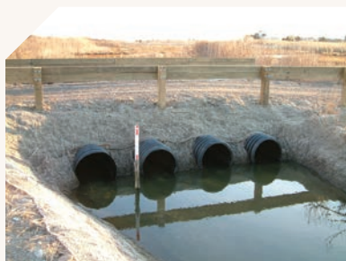
Repaired culvert at Allens Pond Wildlife Sanctuary
